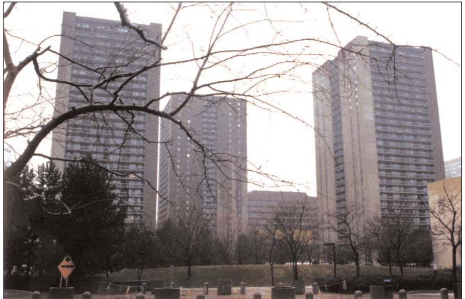
View of the project
